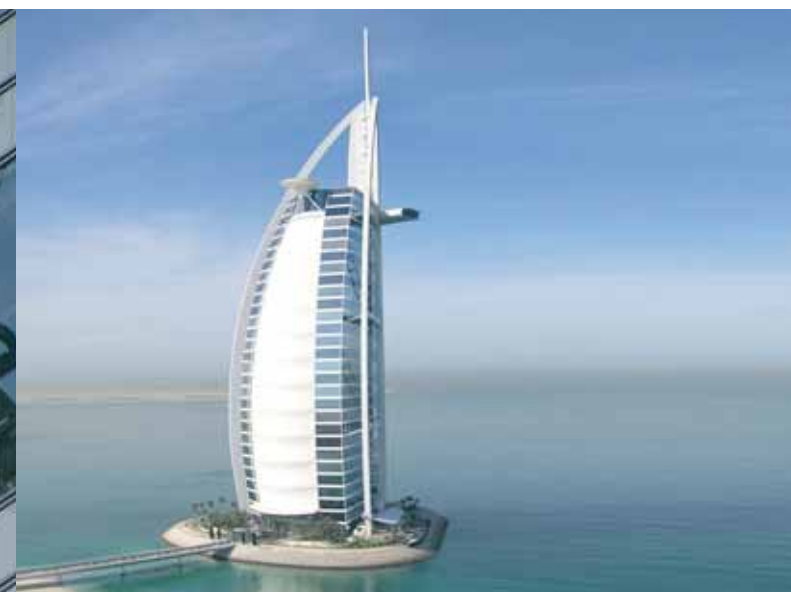
A feasibility study was prepared for the Burj al Arab in Dubai, UAE.
